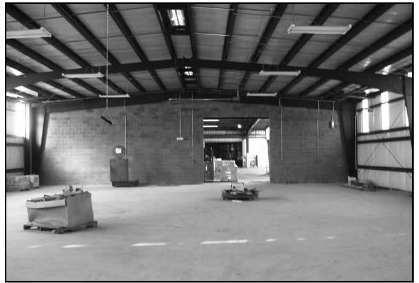
A view from inside the new warehouse
